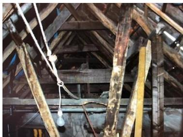
The most significant part of this restoration project was re-roofing. An exhaustive structural survey was conducted, and every roof member was catalogued by age, condition, and structural integrity. The medieval wall plates were retained and repaired in-situ and new oak trusses and purlins
